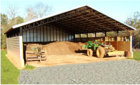
NRCS designed Waste Storage Facility (Litter Barn)
