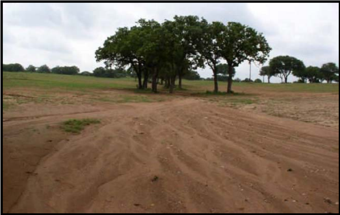
Critical area shaping followed by reseeding of severely eroded area
