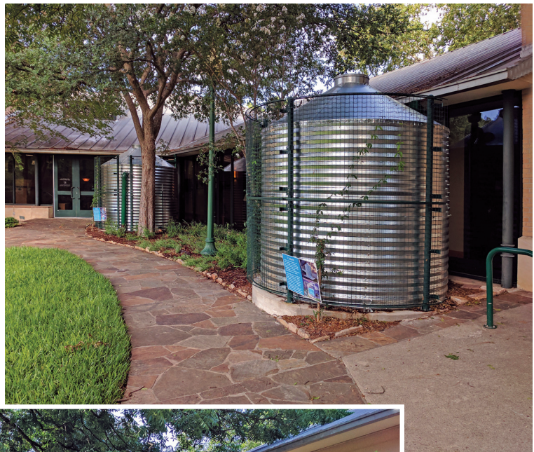
above: Rainwater Cisterns (Source: SARA)
