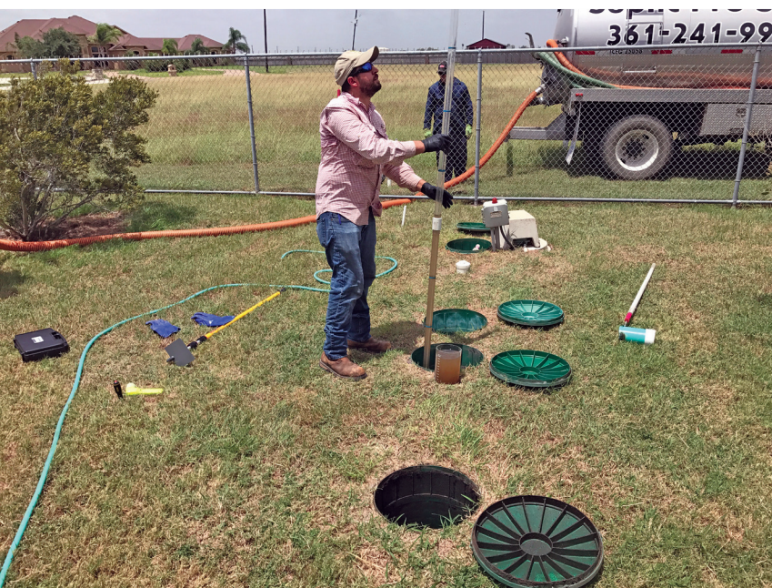
above: Septic System Inspection (Source: Ryan Gerlich, Texas A&M AgriLife Extension)
